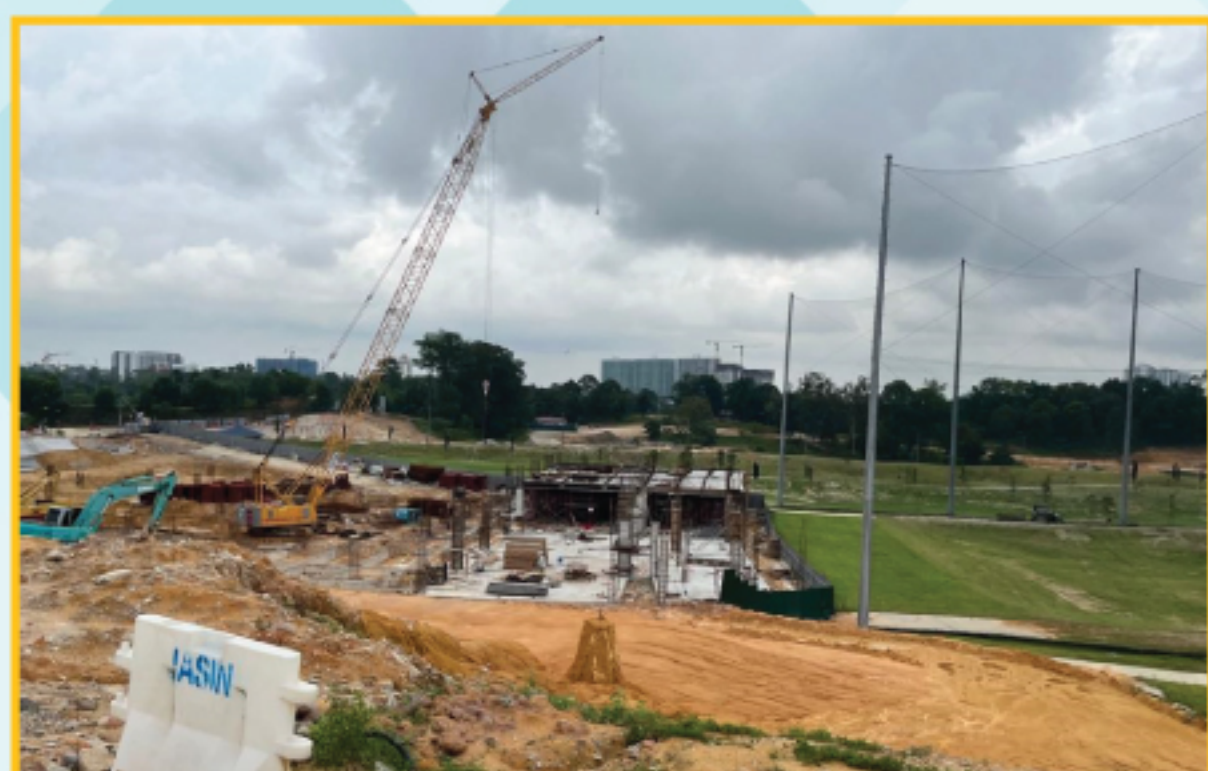
Construction of Driving Range Building.
