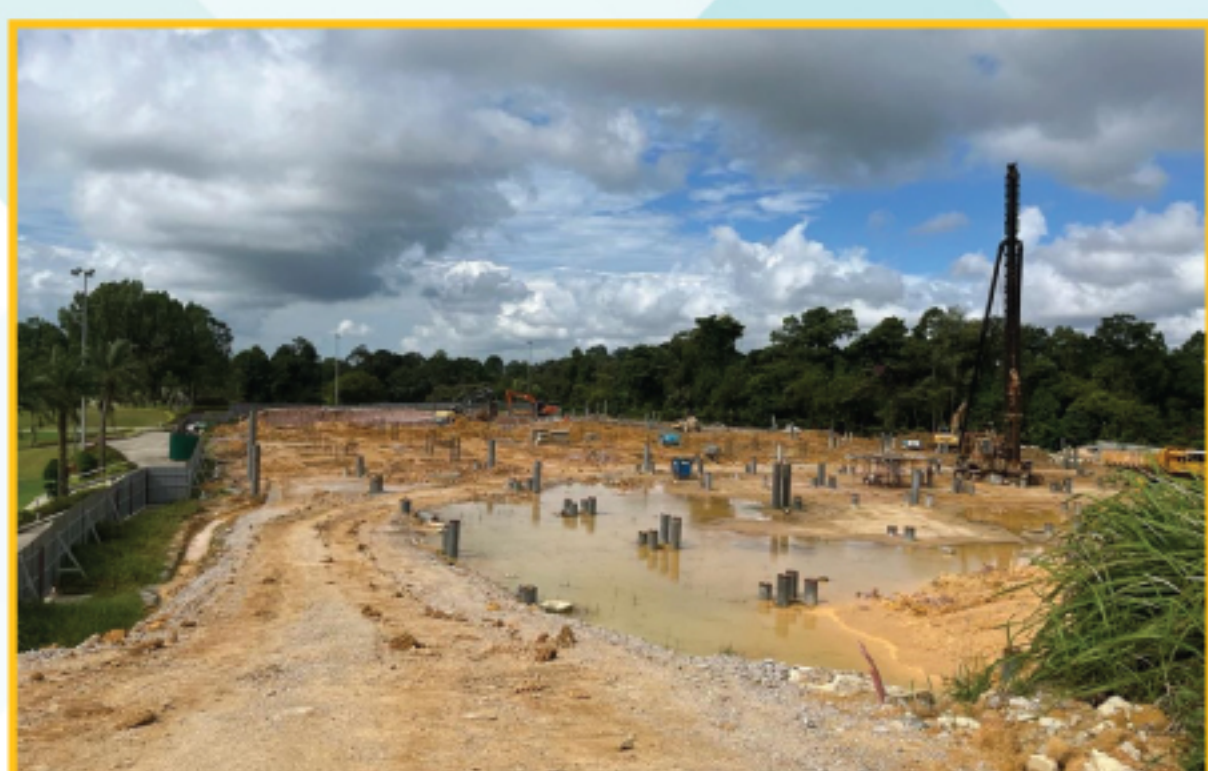
Clubhouse piling works completed.
